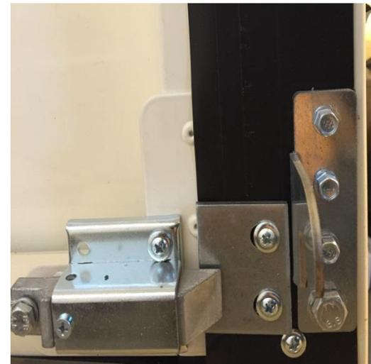
Open the door and fit the spring lower and upper anchor points , as shown -
