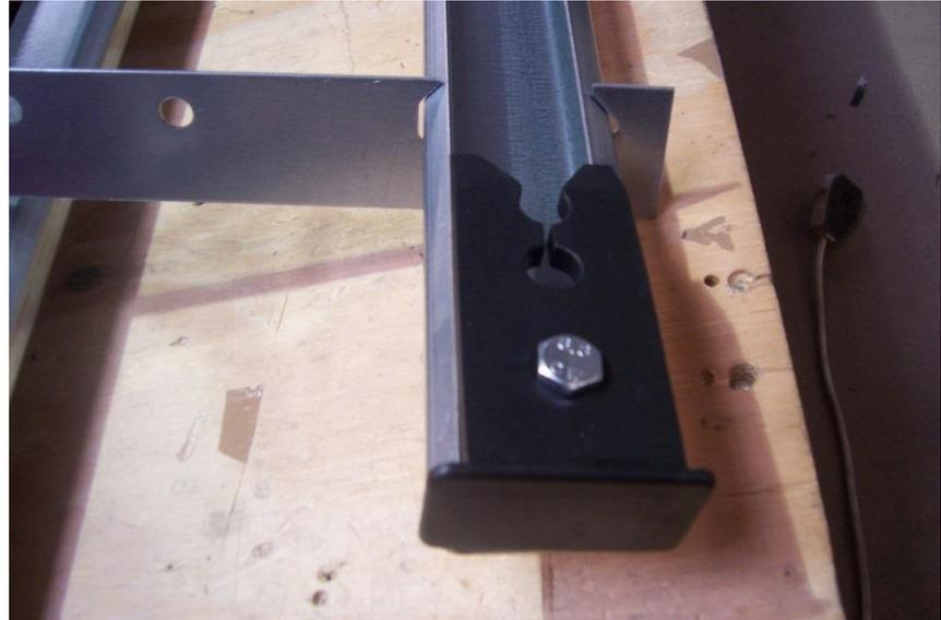
Suspend the tracks from the roof joists , the suspension straps can be cut if required . When fitted you should have a gentle slope from the door end into the garage .(down hill no more than around 20mm )
